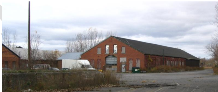
Figure 4.1: Long, narrow warehouse-style brick buildings typify the former DOT “barns” site on the northeast side of the Van Duzee Street Bridge.
