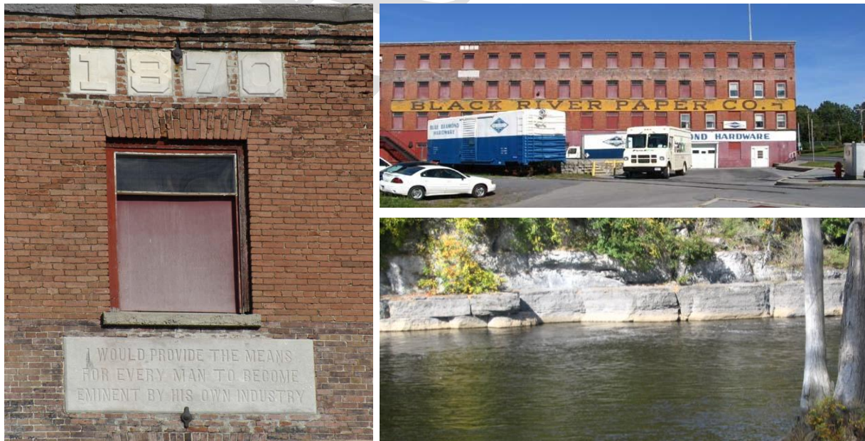
Figures 4.12-14: The Black River Paper Company (right, top) is one of the most visually prominent buildings in the area, and offers substantial adaptive reuse opportunities. These buildings back up to an exceptional stretch of the Black River (right, bottom) that features limestone shelves and cliffs and calmer water currents.
