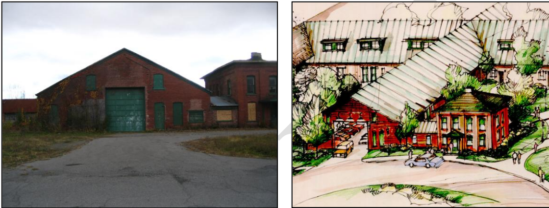
Figures 4.3 and 4.4: The Van Duzee Street Barns current garage entrance (left image) compared to a rendering of potential future interior parking entrance and reception area to the right (right image).
